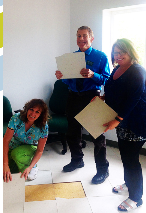
Management Team members happily begin the demolition of the Raymond Clinic.
